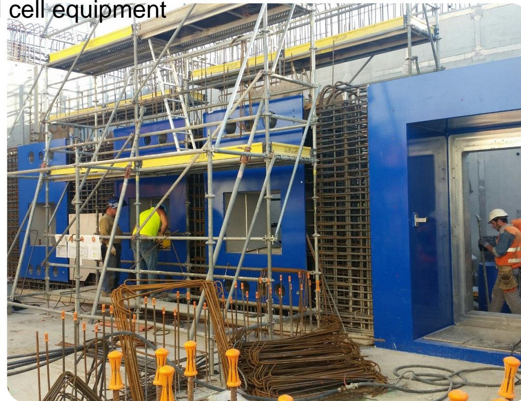
➤ Equipment installation before concrete pouring
