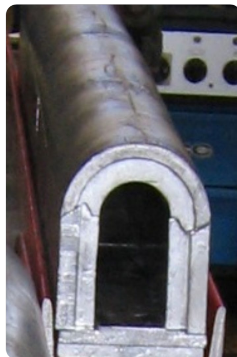
➤ Piping lead shielding
