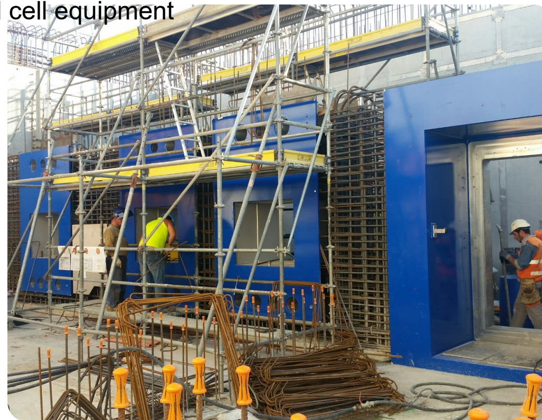
➤ Equipment installation before concrete pouring
