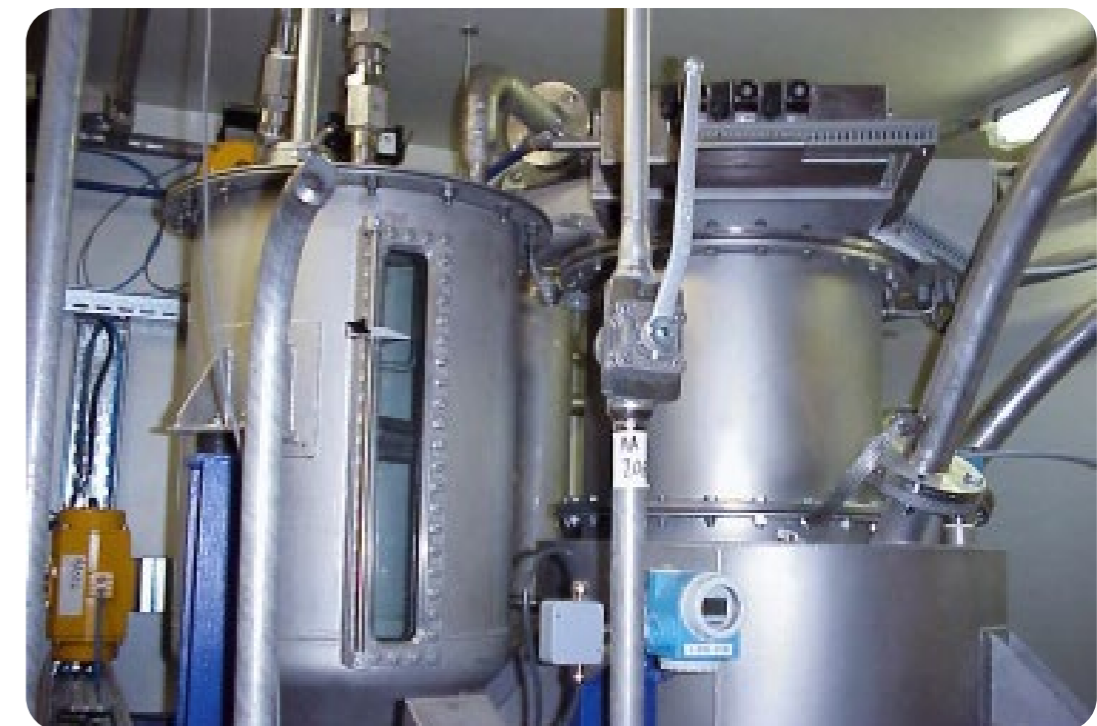
➤ Process de cimentation
